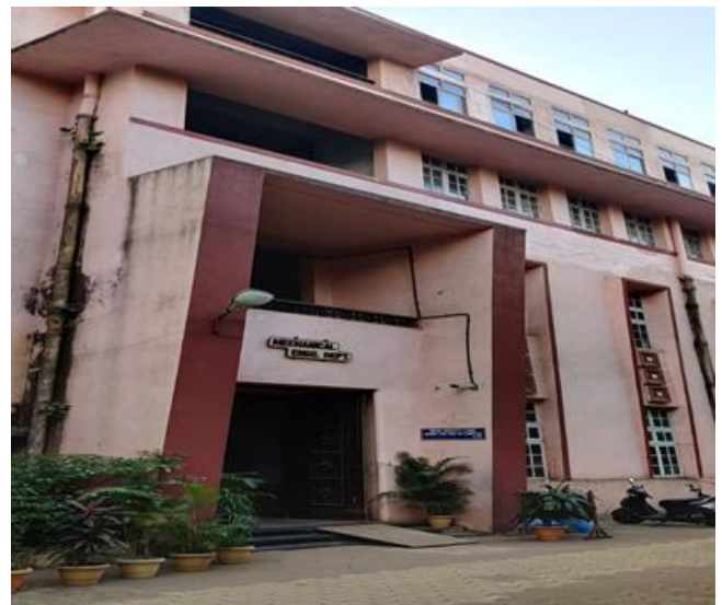
Figure 2: Mechanical Engg. Department building, VJTI
